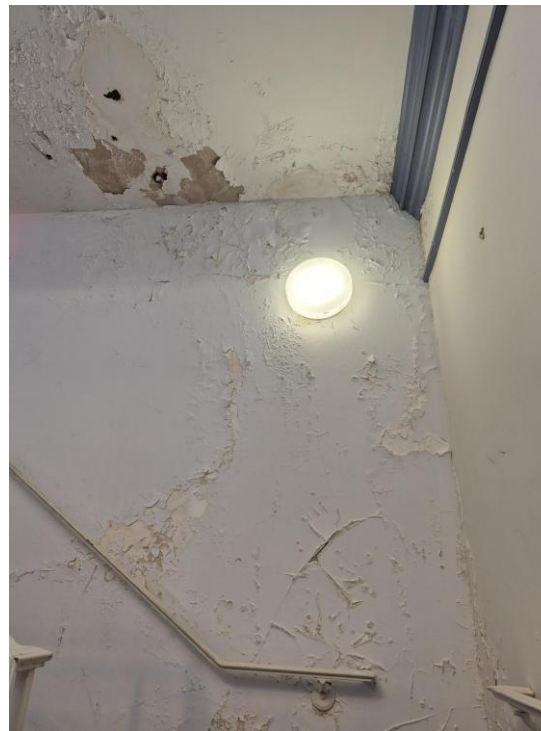
Plaster repairs to prevent water intrusion at the County Courthouse
